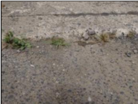
Figure 9 Peeling in pavement
