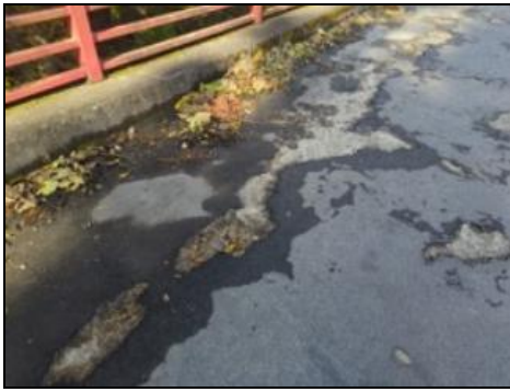
Figure 9 Peeling in pavement
