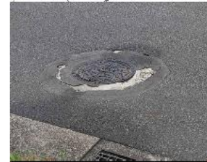
CWA 13 : Renewing or height modification of manhole cover and surrounding asphalt.
