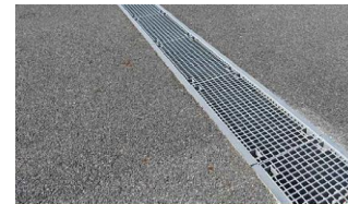
CWA 1 : Replace U-Drain cover with closed cover, or temporarily close while allowing drainage capability underneath.
