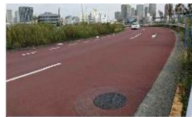
CWA 10.2 (Option to 10.1) : Realignment the Median Island only. Turning lane to be extended. Re-asphalting of this area necessary to local road standards. Possible Road Structure: 30cm subbase; 8cm asphalt base course, 4cm binder course, 4cm wearing course.
