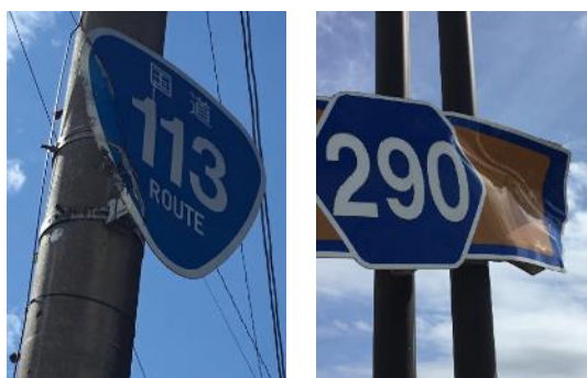
Fig.9 Photograph example of transformation of the road
